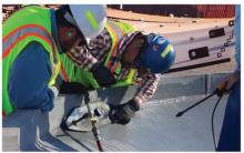
1. Spray area to be vacuum tested with a soapy water solution for better seal and to create bubbles revealing any weld failure locations.
